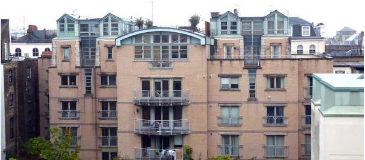
View of roof area from adjacent roof top.
