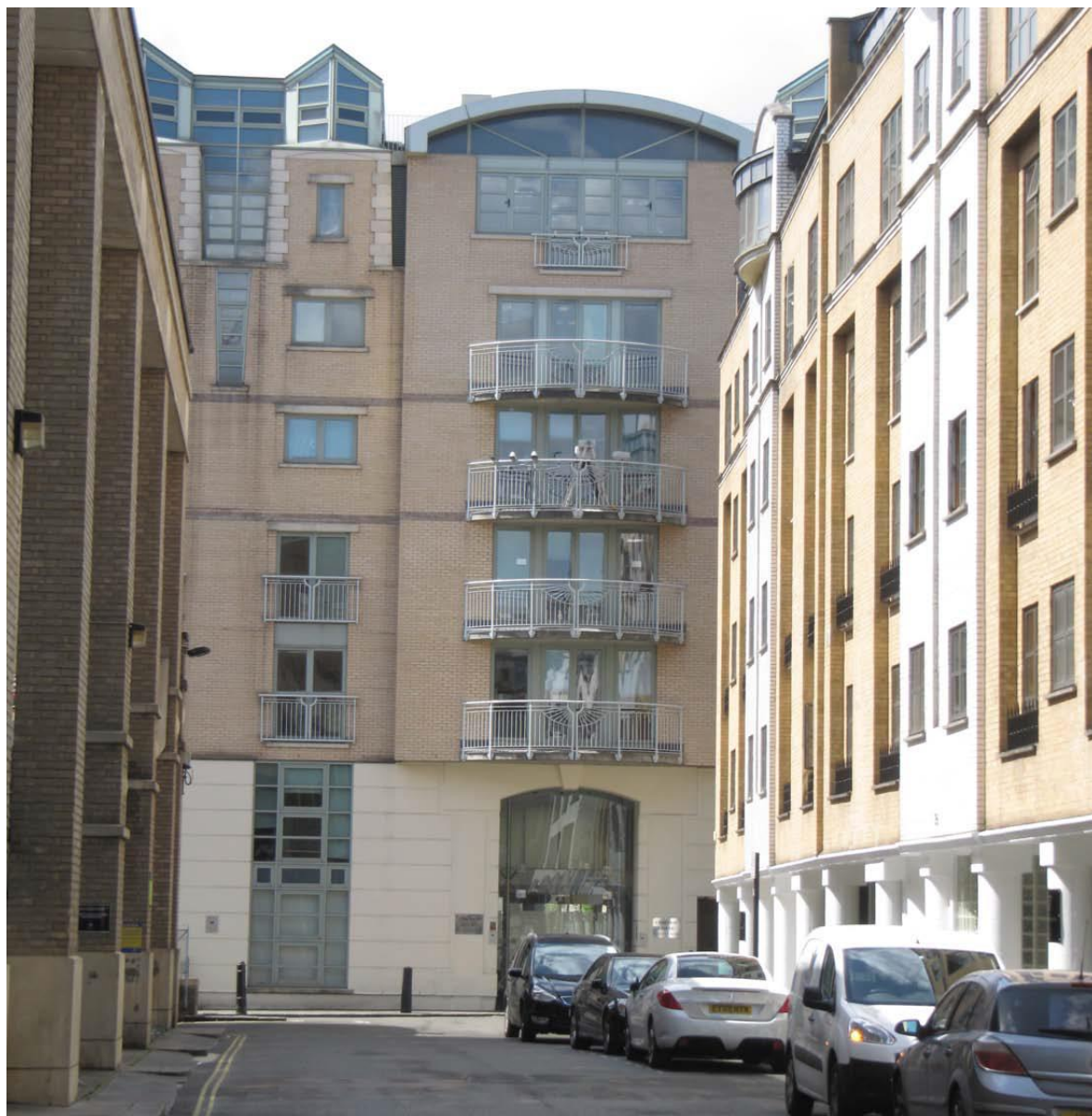
Redan Place View of Building
